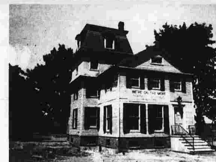
136 NEW LONDON TURNPIKE across from the Post Office
